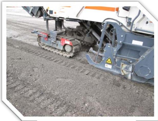
*Milling/Pulverizing Asphalt in Place*
