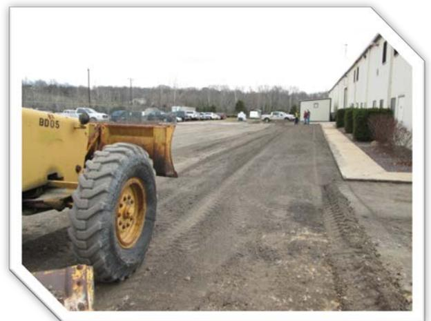
*Grading 1" minus pulverized material*
