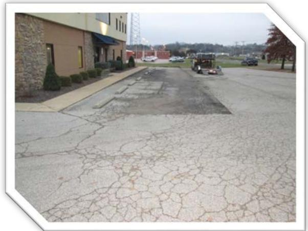
*Existing Parking Lot Prior to Milling (lots of spider cracking!)*
