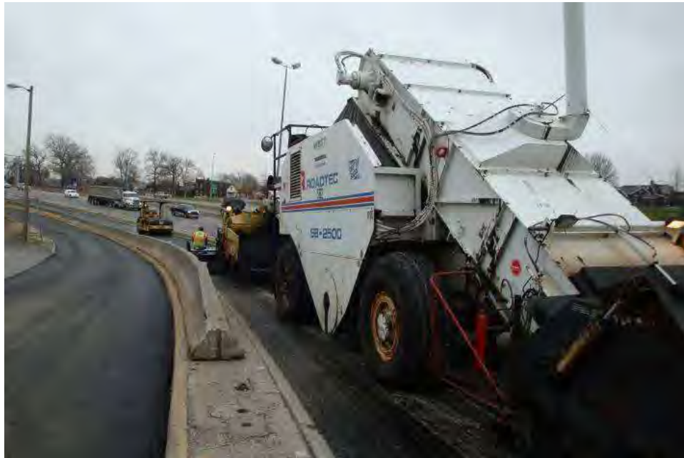
FIGURE 6 Interstate 70 12.5-mm NMAS WMA RAP and RAS Cold weather paving at 23° F (-5°C)
