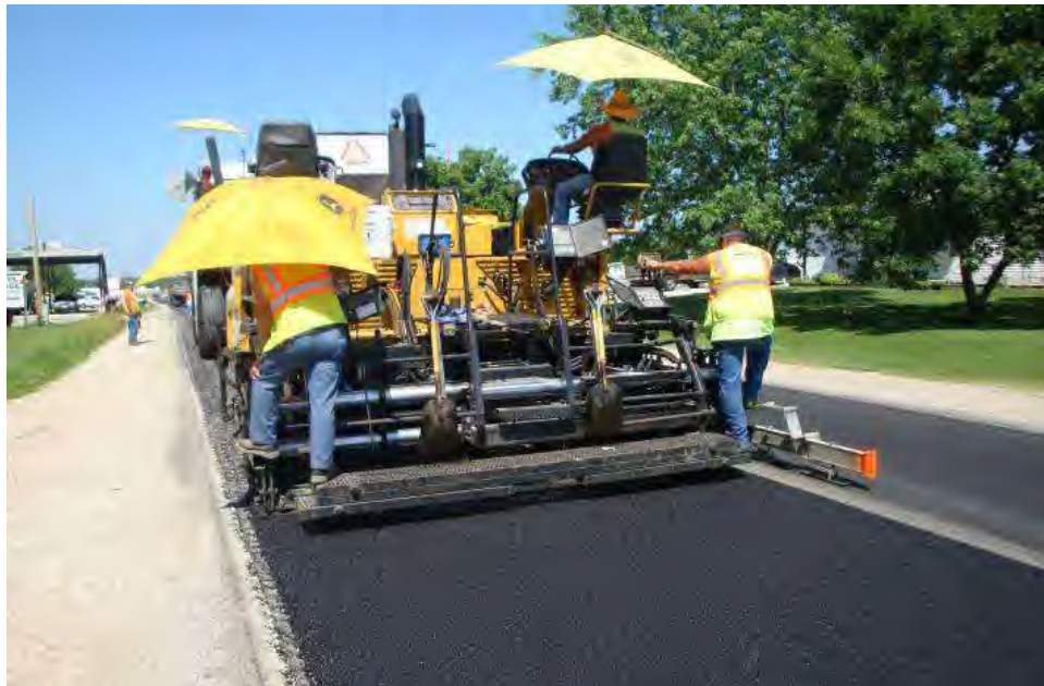
FIGURE 3 Route 50 Gasconade County 12.5-mm NMA S WMA RAP and RAS Pavement
