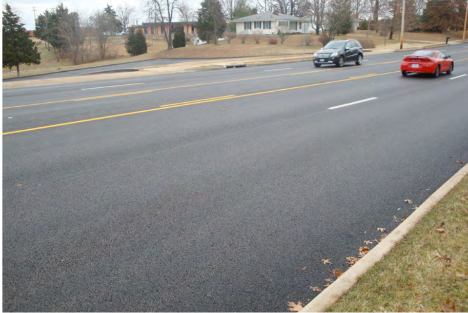
FIGURE 2 Warm Mix UBAWC St. Louis County, MO.
