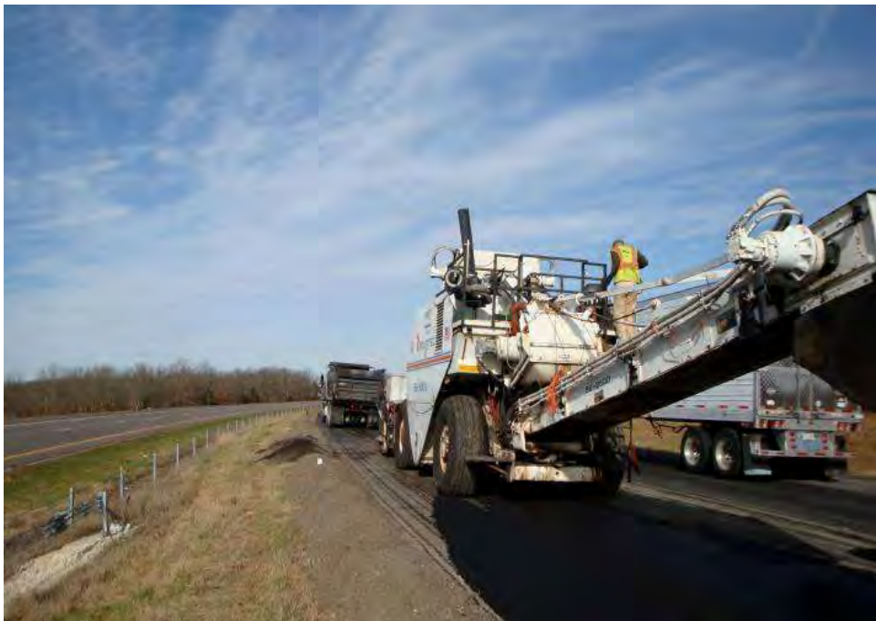
FIGURE 5 Interstate 44 12.5-mm NMA S WMA RAP polymer-modified asphalt pavement
