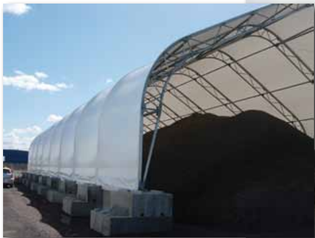
Covering stockpiles helps keep moisture to a minimum, which reduces drying times and temps, thus reducing the risk of blue smoke generation. Photos courtesy of Murphy Pavement Technology, Chicago.
